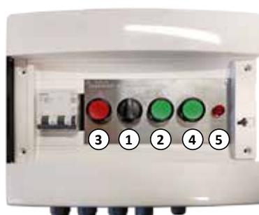
① The MAINTENANCE / NORMAL MODE switch allows to shift from normal mode to maintenance and vice versa; every time you shift from maintenance to normal mode it is necessary to perform a reset by pressing both up and down buttons for more than 3 seconds.
